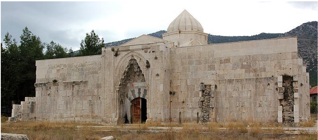
Susuz Han, on the Antalya-Burdur road, showing unadorned walls and entrance decorated with muqarnas and ablaq.
