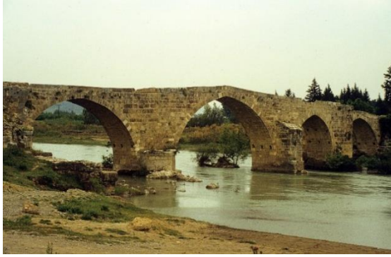
The multi-span Köprüpazar Bridge, 13 th c.
