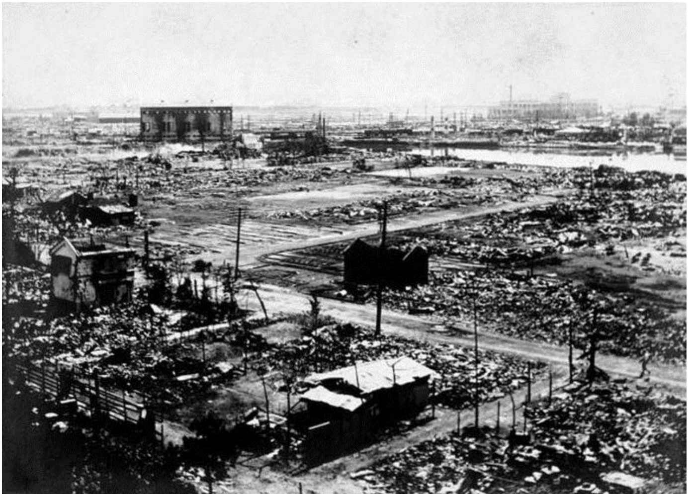
View of central Yokohama following the catastrophic 1923 earthquake (Wikipedia)
